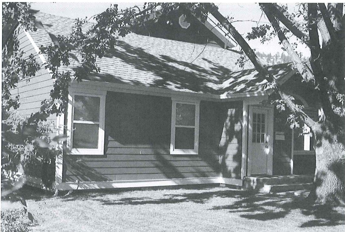
Fig. 20 - 524 Oxford Avenue (from front)
