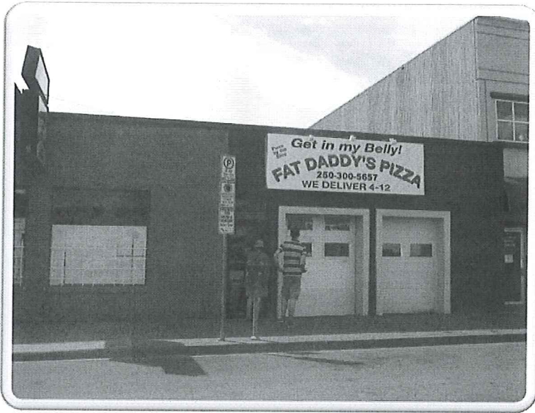
< FIG. 10: 265 (left) and 269 (right) Leon Avenue. This building once housed Jung Shoe Repair (265) and Kwong Sing Laundry (269). The one-storey concrete block building was built in the late 1940s.
